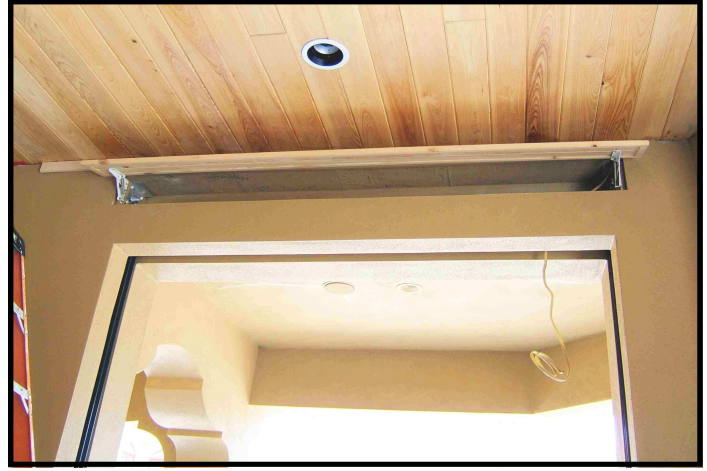
(pictured above) RECESSED: Hood or roller assembly recesses into pocket. Tracks and u-channel are hidden in walls.
